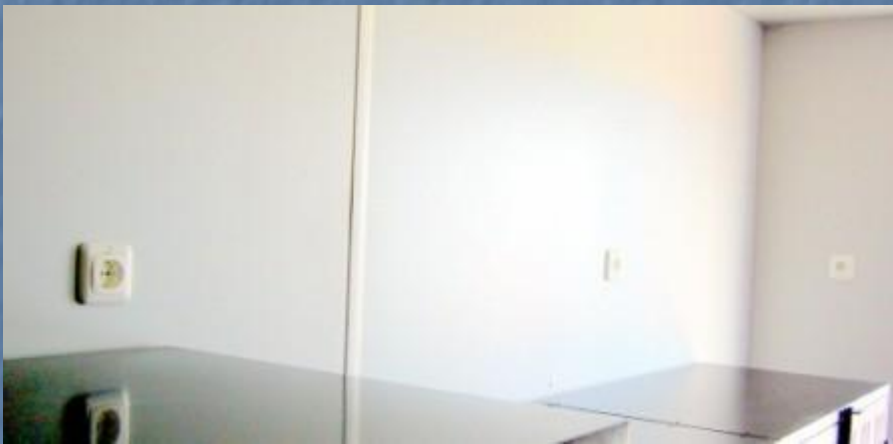
Walls Insulated & Paneled including Outlets
