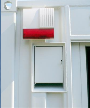
Siren & Strobe with Anti-tampering Switch
